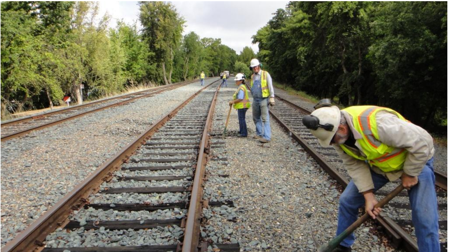
The Team deploys along the Miller Park Siding
