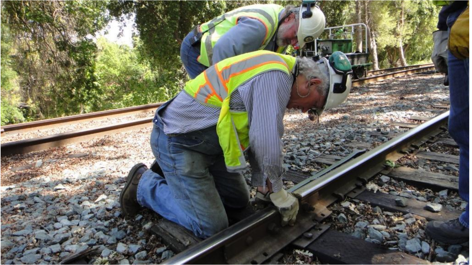
Frank and Steve put the new bolts in place
