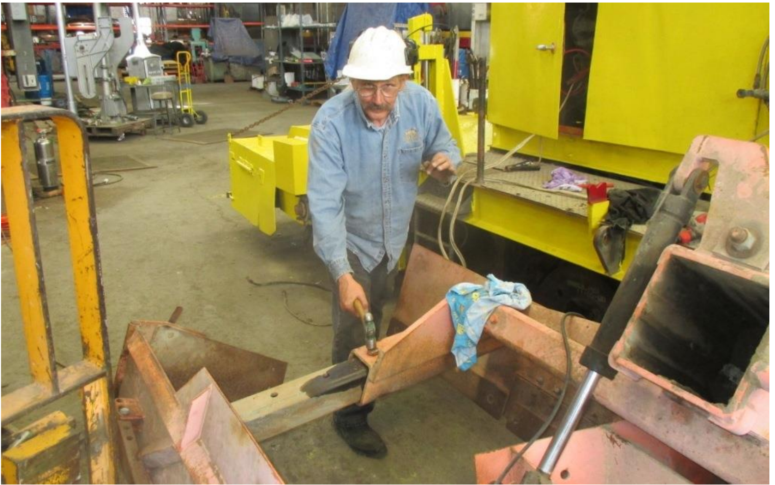
Fred un-seizing bolts to extend the regulator's wing-box
