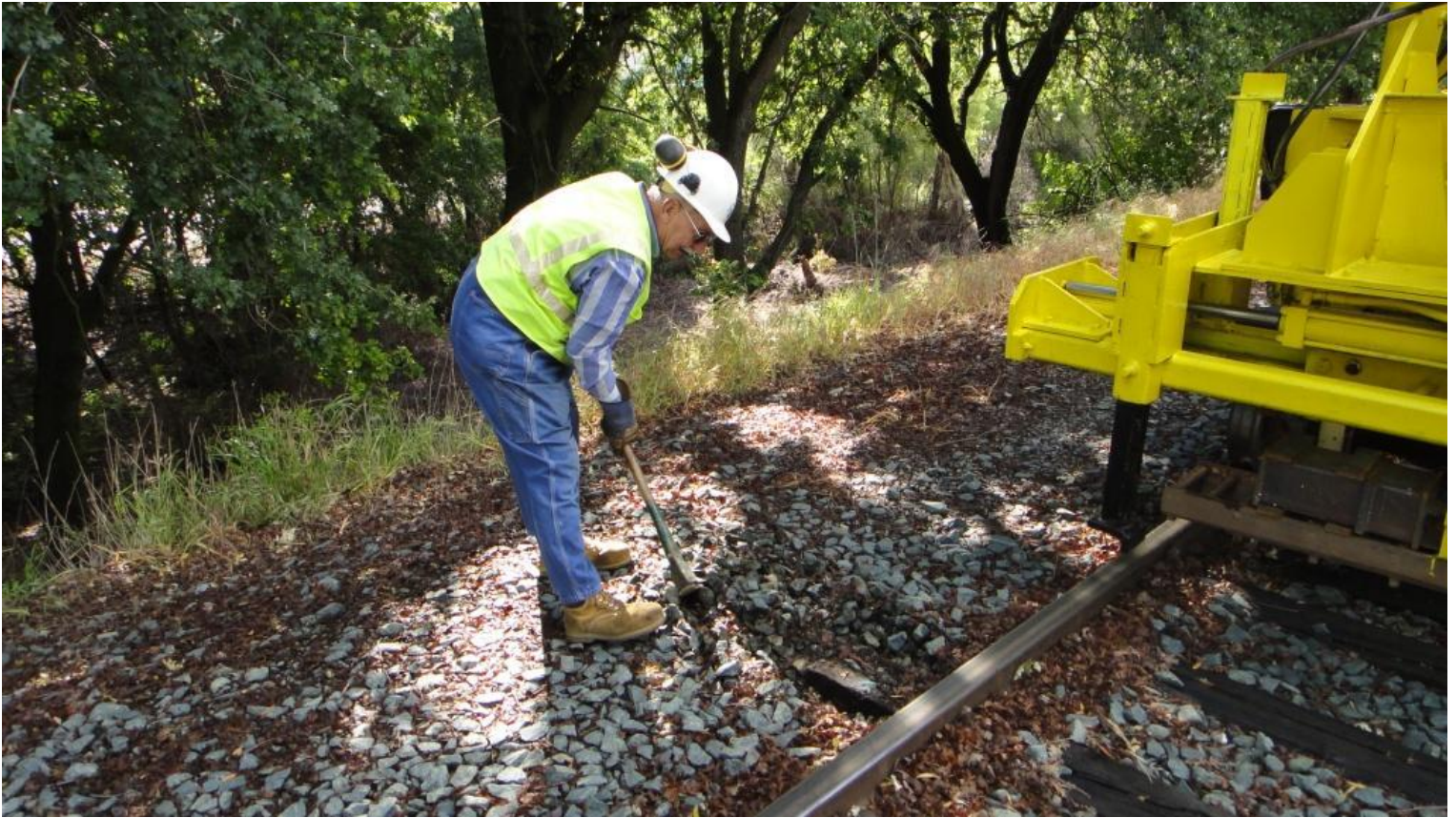
Clem digs out the end of a tie for the 125 to grab
