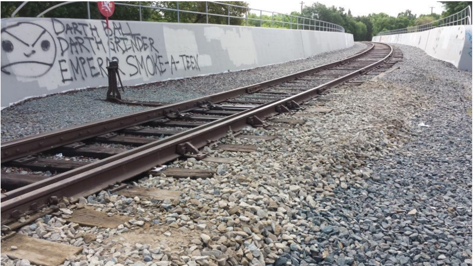
The new west-side brakeman landing strip at Switch 20
