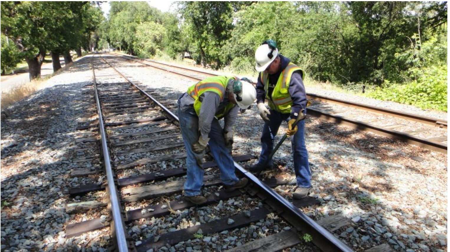
Steve holds the bolt against the rail with his foot while Ed removes the nut
